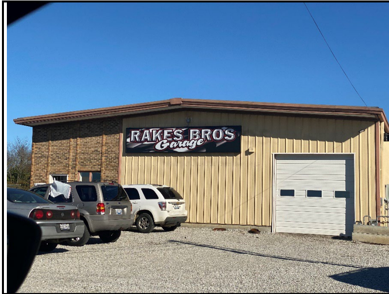
Mechanic Shop located along KY 55
